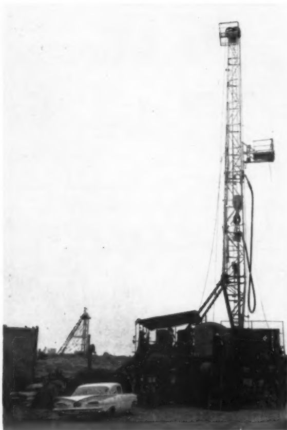
SECTION 17 ventilation shaft was drilled first. Here is Rayco Drilling Company's Rig No. 3 making hole with big bit.
